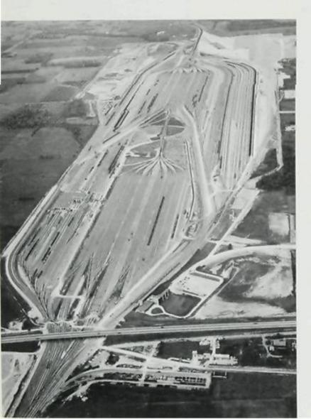
Freight accounts for most of the railway traffic and the greatest recent advances in railroading technology have undoubtedly been those related to the sorting and segregating of freight cars. The modern "hump yard" uses radar computers and closedcircuit television and is heavily automated. The new CN yard at Toronto covers 1,000 acres, has 156 miles of track and can process 6,000 freight cars daily.
